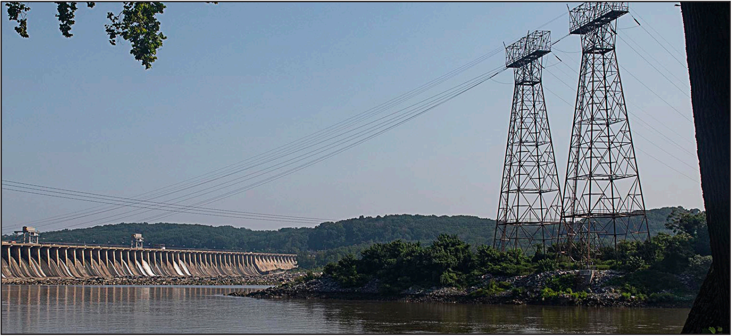
Photo Courtesy of Conowingo Dam, Tony DeYoung
